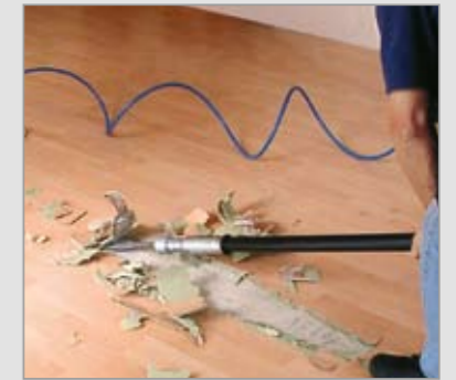
Floor coverings stripped with ease
