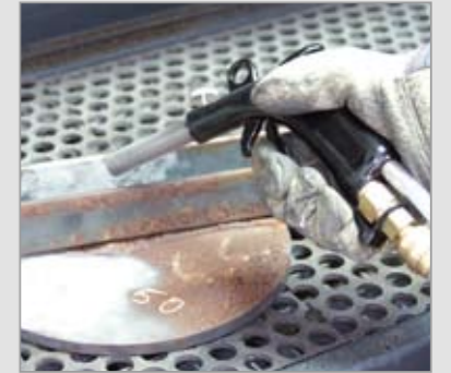
Sand blasting – fast and effective
