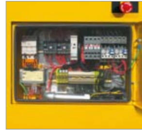
Control cabinet Completely wired; control panel includes operating hours counter and mode selector switch.
